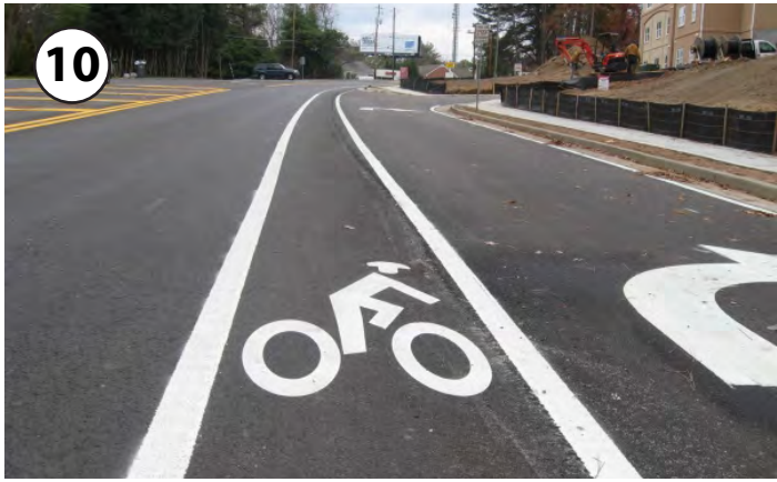
Restriping traffic, bicycle, and parking lanes that have faded can assist school traffic operations.
