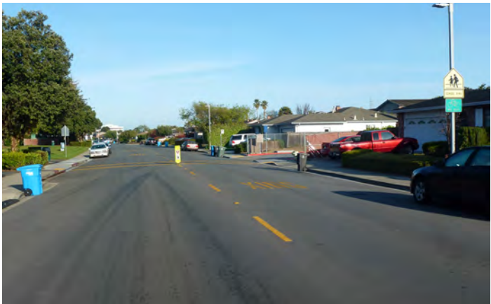
Uncontrolled transverse crosswalks can be difficult for motorists to see without additional crossing treatments.
