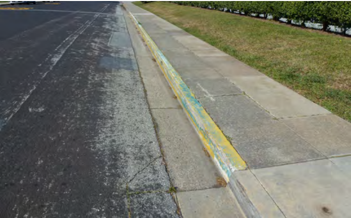
Faded curb paint does not clearly communicate parking restrictions on the curb.
