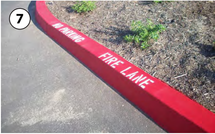
Red curb paint delineates areas where parking is prohibited.
