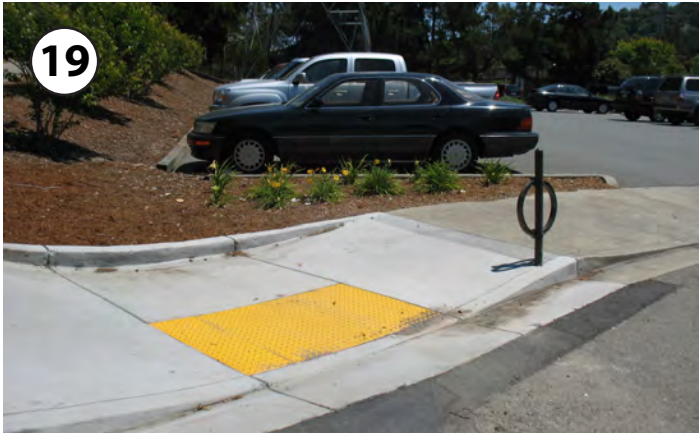
Curb ramps provide access to disabled pedestrians and parents walking with strollers.
